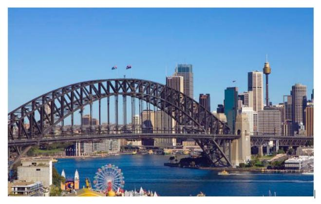
The lower arch of the Sydney Harbour Bridge can be modelled using the equation:  $y = -0.00188(x - 251.5)^2 + 118$
